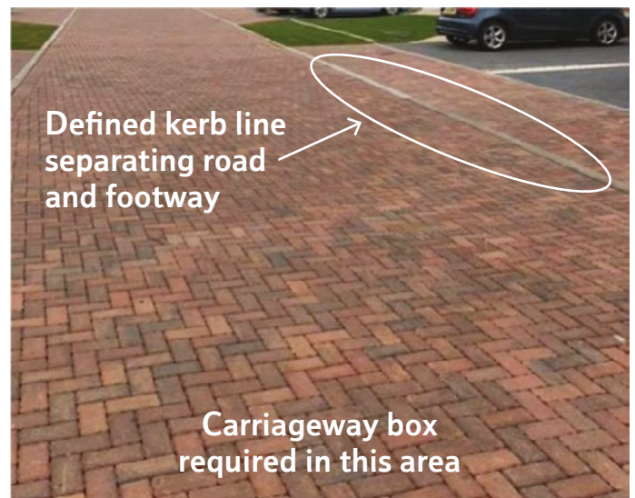
Example of a defined kerb line on a shared surface
